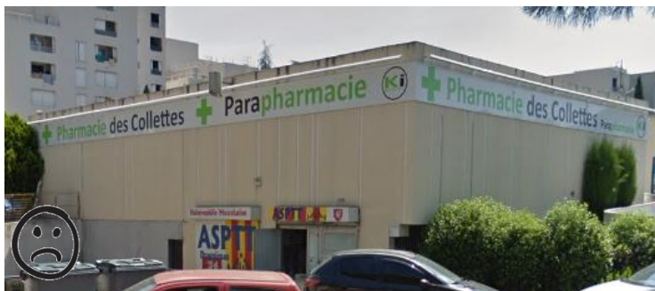
99. Centre commercial des Collettes – Ch. Ste Barbe
